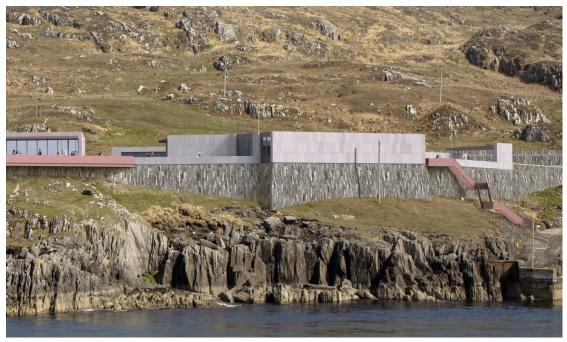
Plate 2.11 Proposed stone-clad screening walls.
